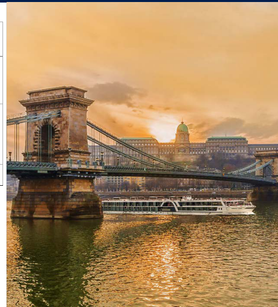
Budapest chain bridge
