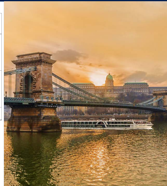
Budapest chain bridge
